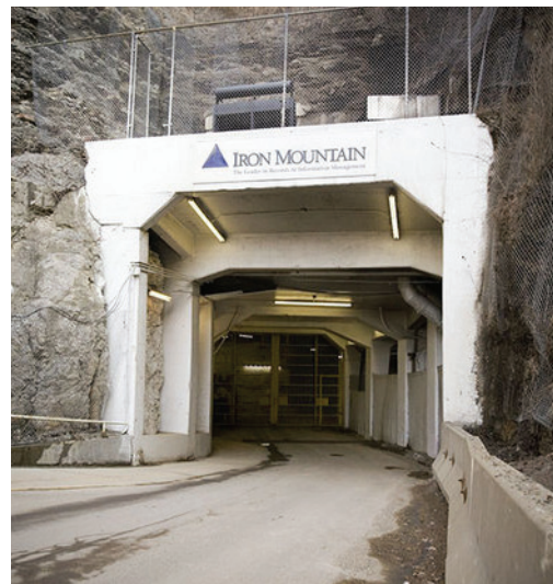
Entrance to an Iron Mountain underground facility.
